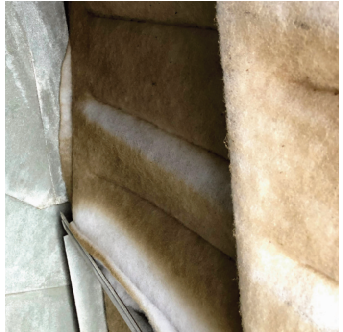
Figure 76. Dirty air filters
